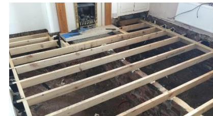
Timber suspended floor- used in smaller buildings
