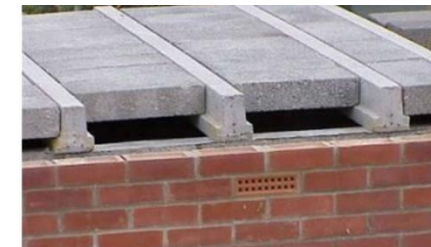
Beam and Block floor- used in larger buildings
