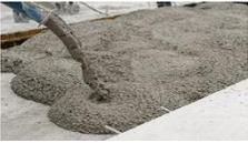
**Concrete-** strengths range from 8 N/mm<sup>2</sup> to 60 N/mm<sup>2</sup>
